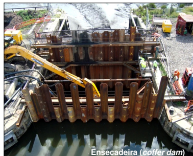
Ensecadeira (coffer dam)
