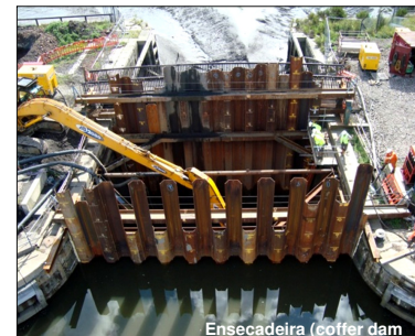
Ensecadeira (coffer dam)
