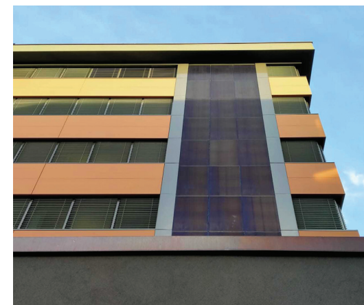
Fig. 1, 2 General view of the building after and before the retrofit of the façade. Source: P. Corti.
