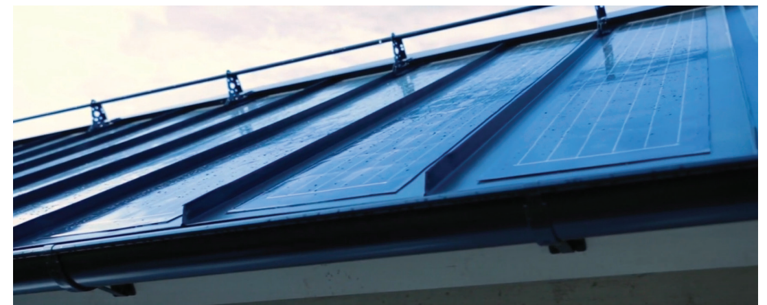
Fig. 2 Detail of the BIPV roof. Source: Midsummer.
