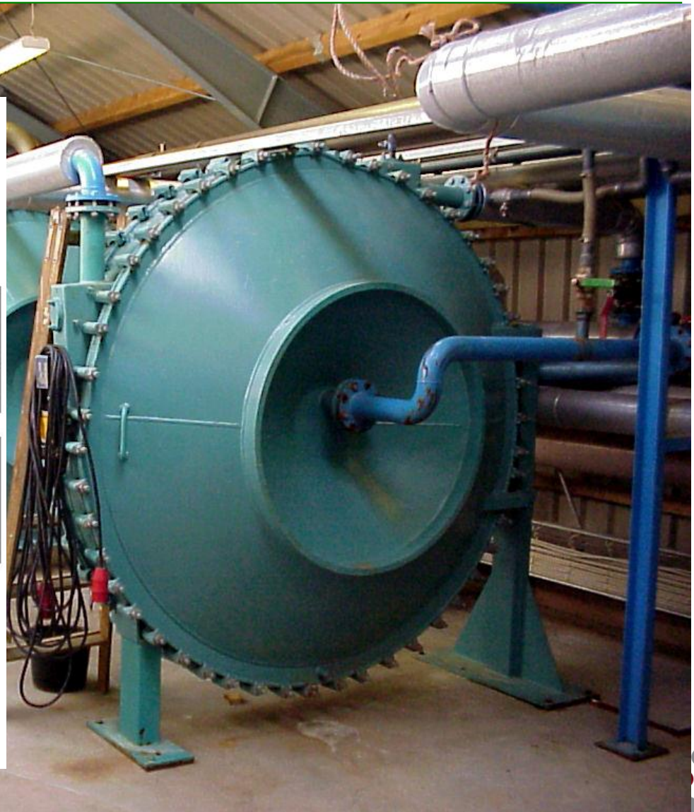
Design of a Sondex spiral heat exchanger
